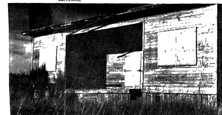
The refrigerator room stand empty. It's windows boarded.
